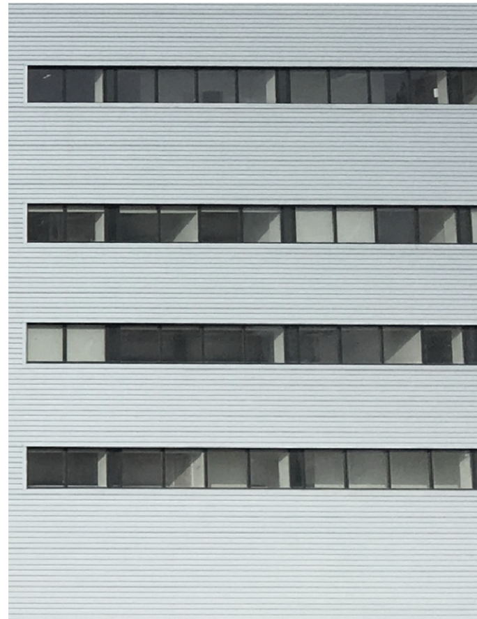
Field Cladding - Cladding Type A Euroclad Elite 55 Reverse Profile Insulated Horizontal Cladding
